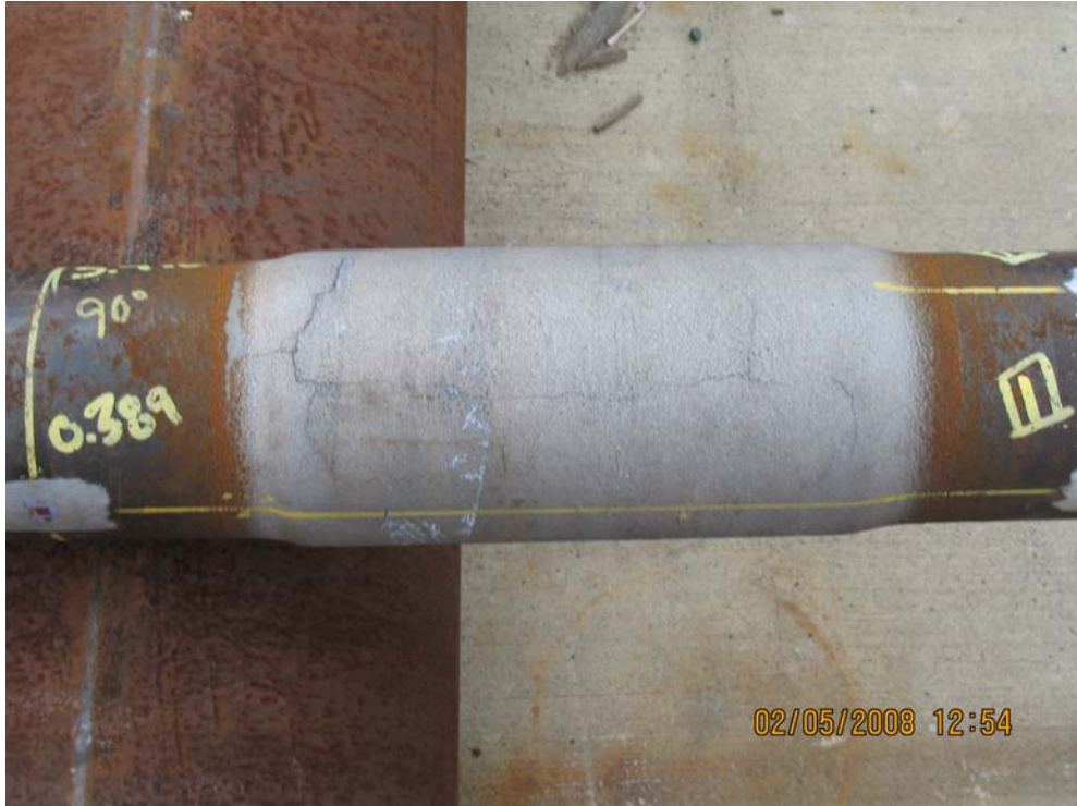
Figure 3 Outboard WearSox band that developed cracks.
